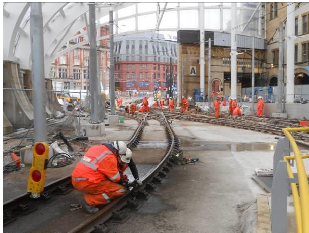
Above and below, large numbers of track workers were needed to have the new stop open for through traffic of trams a couple of days later. Notice the unusual curved diamond crossing in the centre of the picture. Most of this layout is now in regular use.
