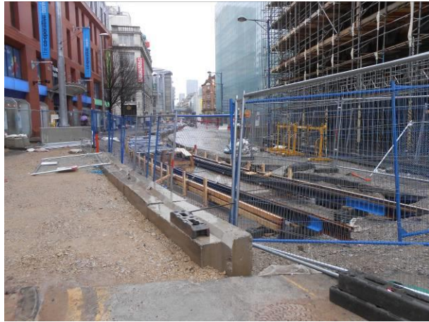
Work on the second city-crossing at Cross Street near Victoria station.
