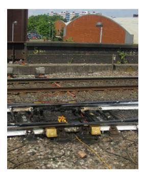
The solution required a lot of hosepipe and a rotary garden sprinkler. This eventually washed the grease off the switches leading them to jam – so an extra greasing was needed as well.
