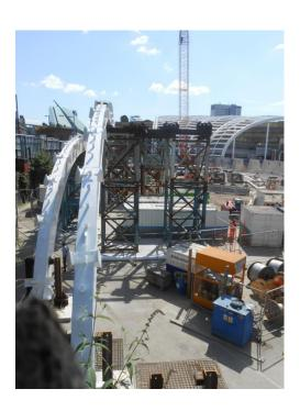
Installation of the elliptical girders to support the new curved roof is progressing well at Manchester Victoria Station.
