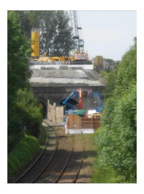
At publication date Lillie has been installed and has disappeared into the hillside. Spoil will be ejected from this end of the tunnel and driven over the top in lorries.
