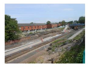
The next photograph shows why. The tracks will have to be slewed to the left (East) to go through the new tunnel, leaving the old smaller tunnel out of use.
