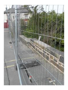
Below the bridge you can see the instruction on the retaining wall. This seems to indicate that the track will be lowered at this point to create more clearance for the OLE.
