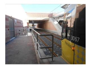
Piecemeal bits of work are taking place to **repair the crumbling brickwork and platform edges** at Eccles Station. A small work compound has been established under the steps to the Liverpool platform. This follows about 50 years of neglect and is part of the increased cost of running an improving railway rather than a decaying one. *Photos by JERayner*.
