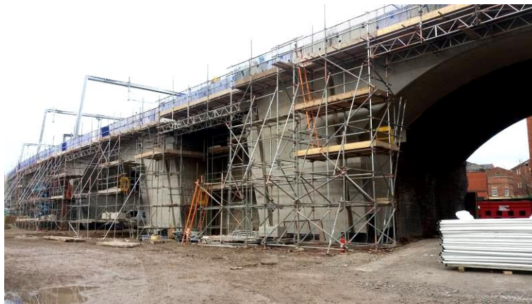
A steel viaduct span is being constructed ready to insert into the viaduct over the Irwell.
