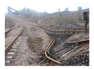
The twisted track at Hatfield Colliery, as a result of the landslip.
