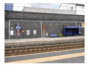
Work has been continuing at Eccles station to install electronic information equipment. Here you can see the ducting introduced on the retaining wall of the Liverpool platform. Note also the new pointing of the brickwork just below the platform edge. Photo:JER
