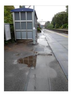
Although the platform for the Manchester trains has received some attention to improve its drainage during wet weather there is still a problem caused by the uneven surface of the platform. One of the resulting puddles builds up in one of the doorways of the further shelter, and even begins to make its way inside.
