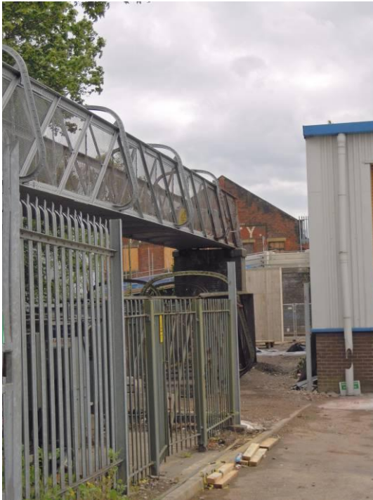
Chadwick's footbridge (four bridges) - photo taken from the Monton side.
