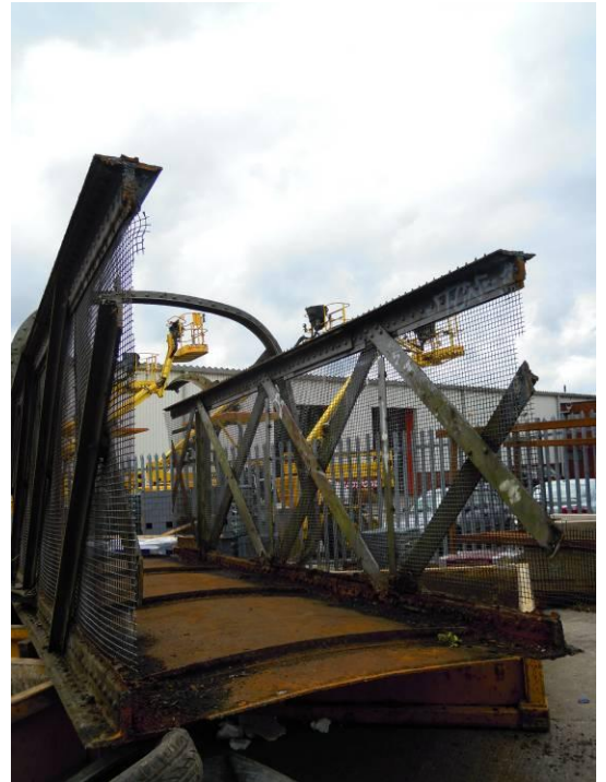
A forlorn section of the old main spans is waiting to be taken away on a scrap lorry. Notice the shallow base to hold a thin layer of tarmac.
